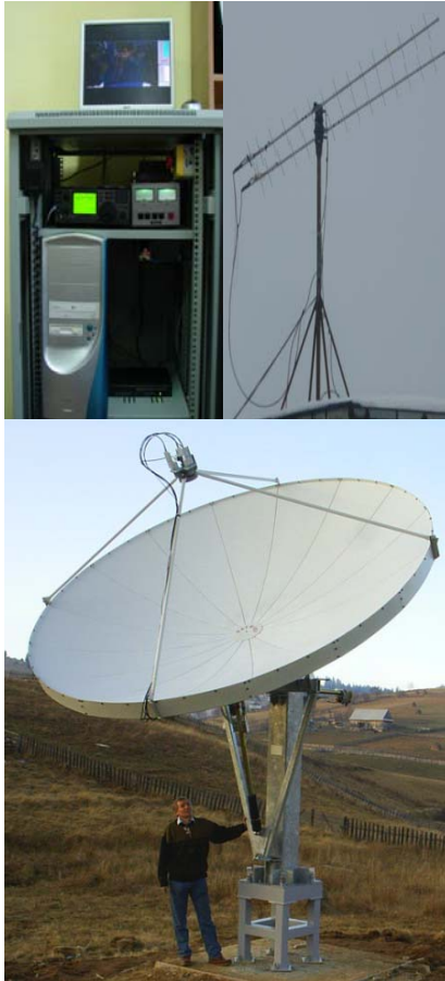
Fig. 10 UHF Control Equipment (up left). UHF antennas (up right). 2.4 GHz Dish (down)
